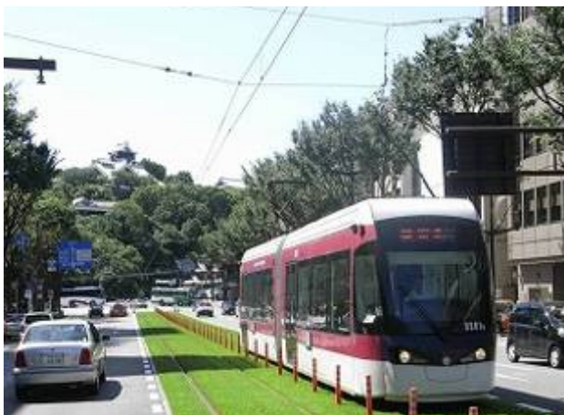
The city promotes tram track turf-laying project
