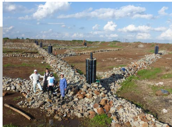
Landfill Site in Kenya that used the Fukuoka Method
