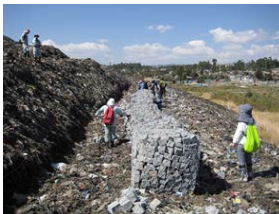
Gabions being constructed by local employees.
