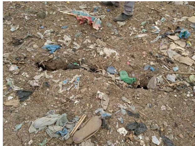
These cracks are the sign of possible collapse.
