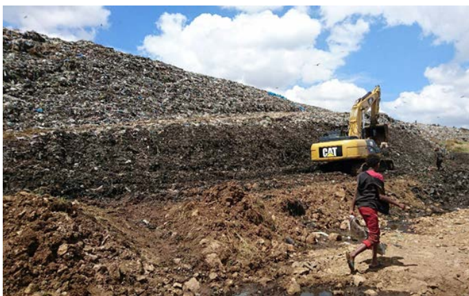
Stabilizing the dump site by using heavy machinery.
