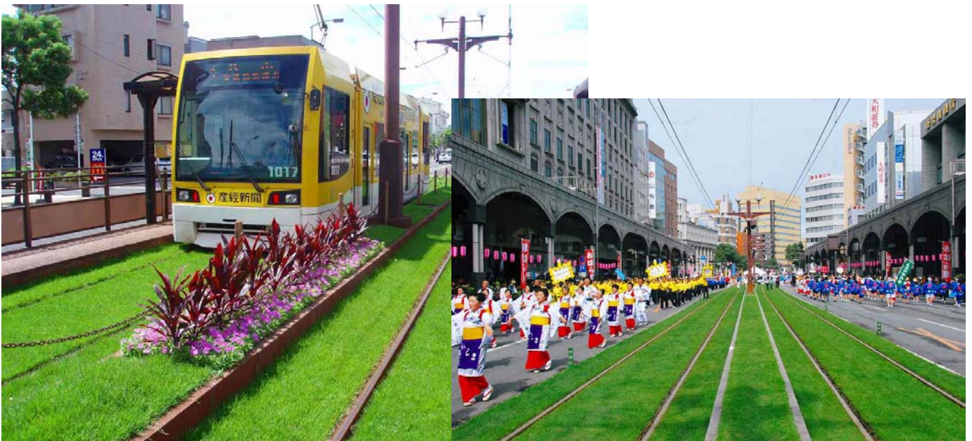
Making major contributions to greening in cities Kagoshima City Tram Track Turf - laying Project (Kagoshima City)
